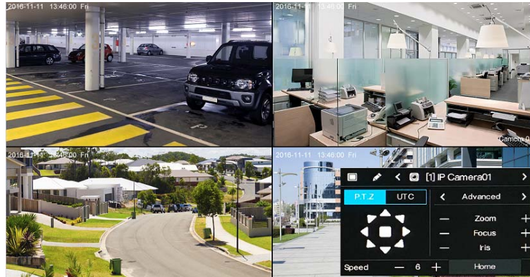
Figure 3-3 PTZ control screen
