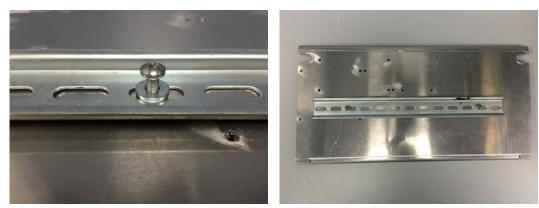
Re-attach the mounting plate to the enclosure and tighten bolts.
