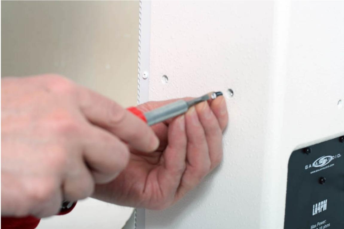
2. Select the appropriate holes in the yoke for the tilt angle desired. Available angles are: 90 degrees (level), 10 degrees or 15 degrees of tilt. (See photo below.) The yoke may be mounted to the wall upside-down or not, to provide upward or downward tilting at both angles.
